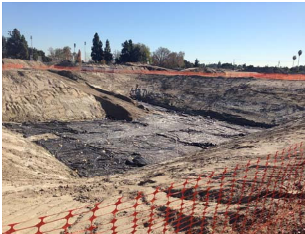
Photo 3 – Final View to Southeast of Ex #35 with Plastic Cover (December 9, 2015)
